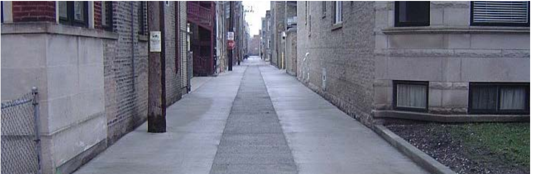
High Albedo Concrete Alley with High Albedo Permeable Concrete Trench
